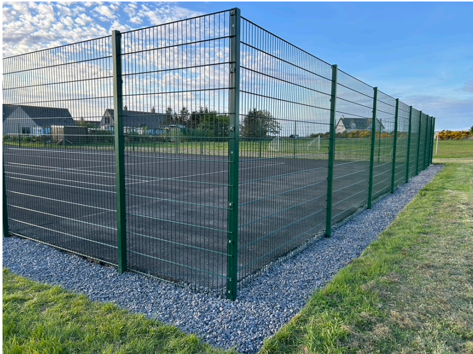
Tennis court resurfaced and new boundary fence
