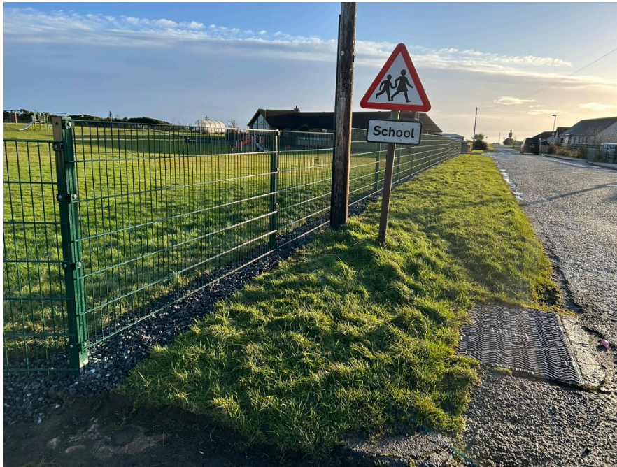
Park boundary fence renewal.
