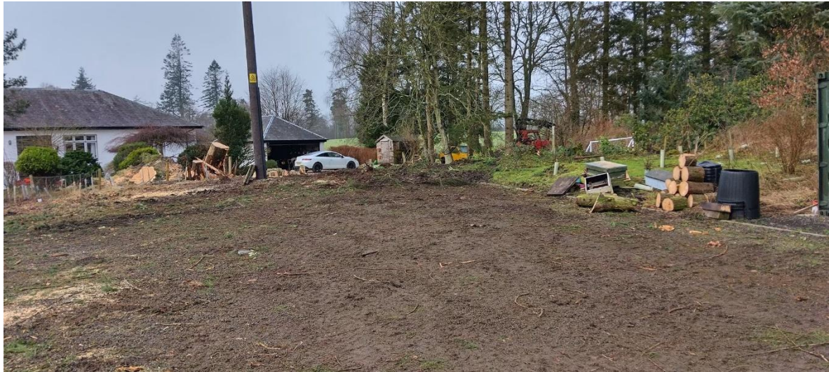
Carpark cleared and new poles up
