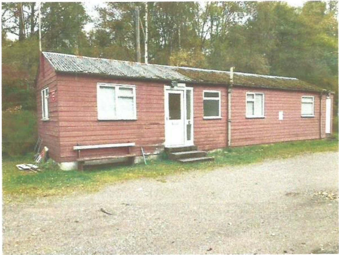
RECREATION ROOM – BEFORE RENOVATION
