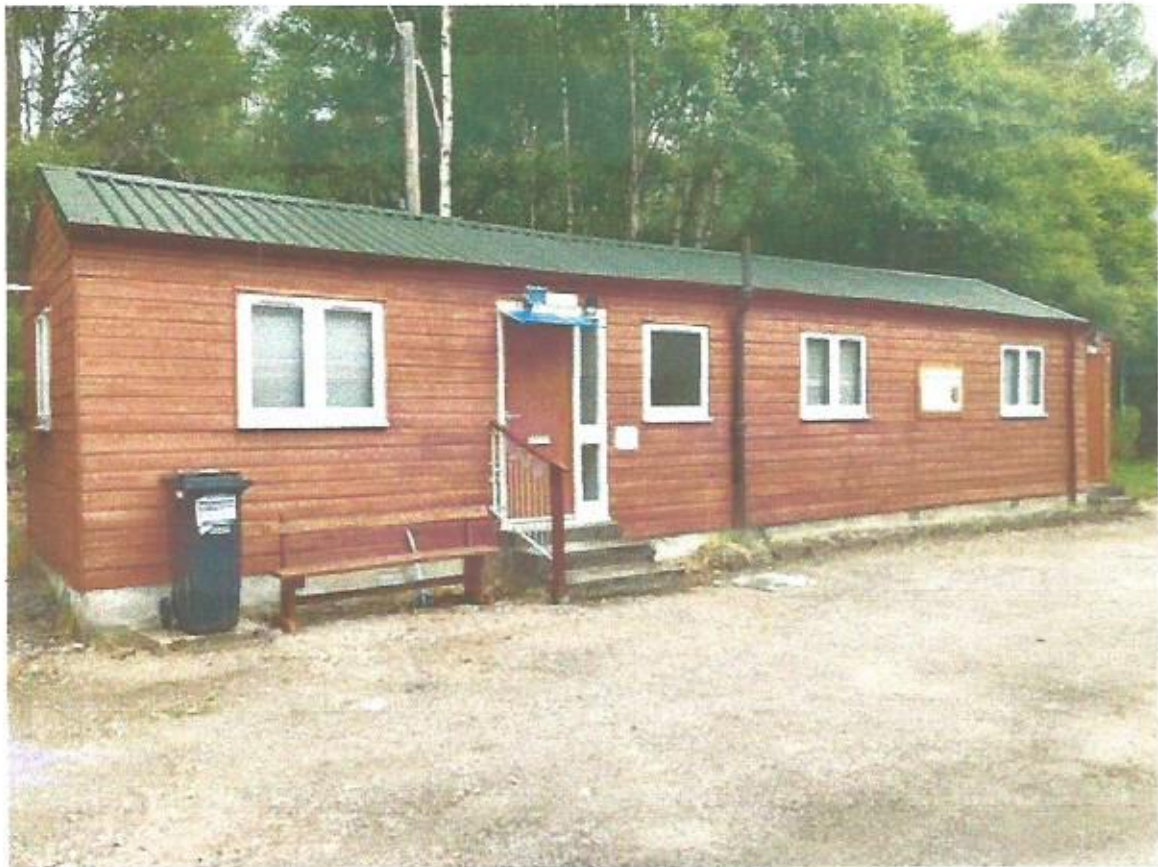
RECREATION ROOM – AFTER RENOVATION
