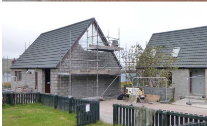
Stucco blockwork replacement works.
