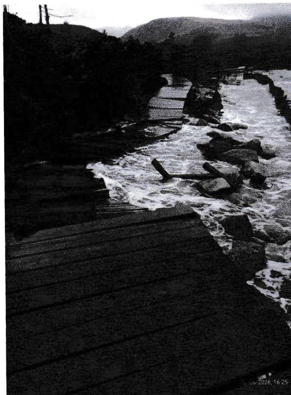
Above: Easterly winter storms have destroyed parts of Fisherman's Walk
